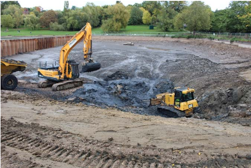
Picture 2 - De-silting Model Boating Pond using excavators
