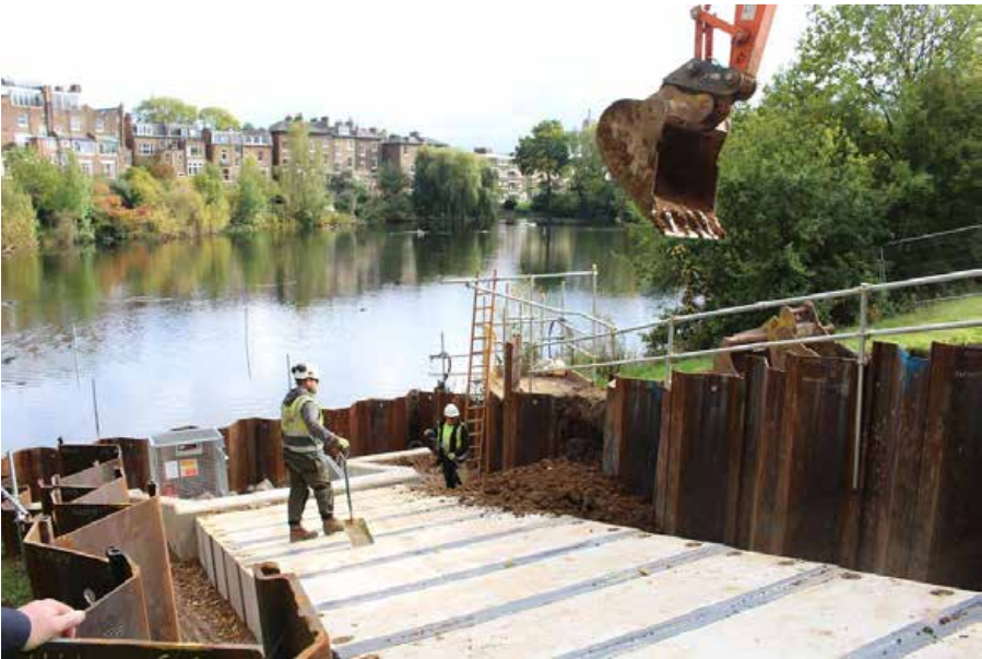
Picture 6 - Works underway building the culvert between Hampstead No. 2 and 1.
