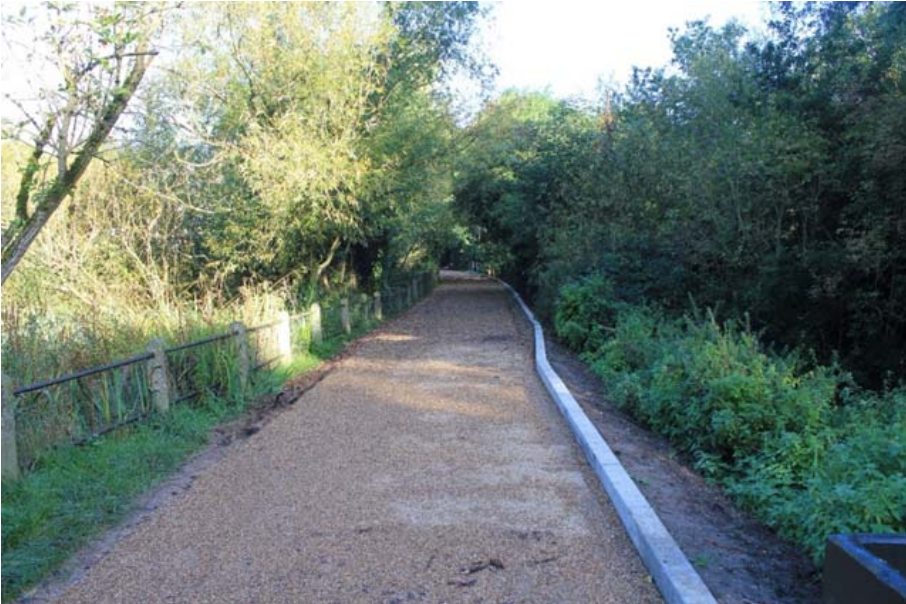
Picture 5 - Completed works at Vale of Health
