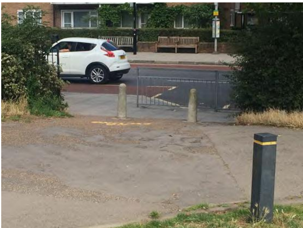
Figure 6 – Replacement of two concrete bollards with wooden bollards (Note 9, appendix 3 - proposed layout).
