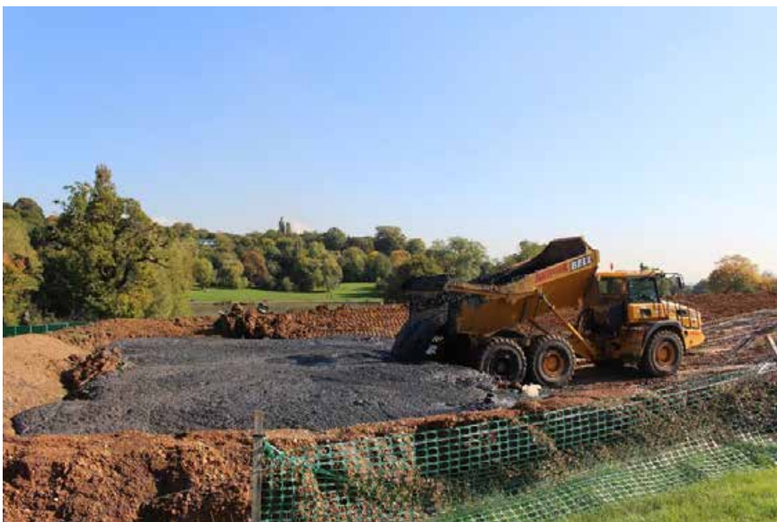
Picture 3 - Silt deposited to dry out in work compound next to Model Boating Pond.
