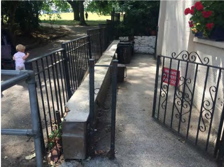
Figure 1 – Remove metal railing and replace with wood post and rail. (Note 1, appendix 3 - proposed layout).
