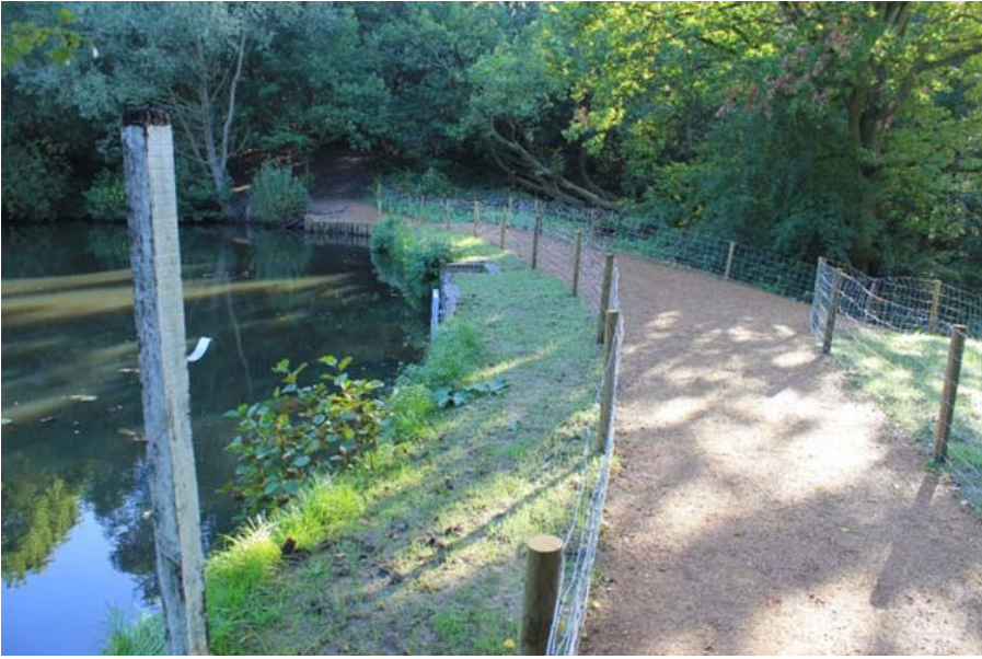
Picture 4 - Completed works at Viaduct Pond
