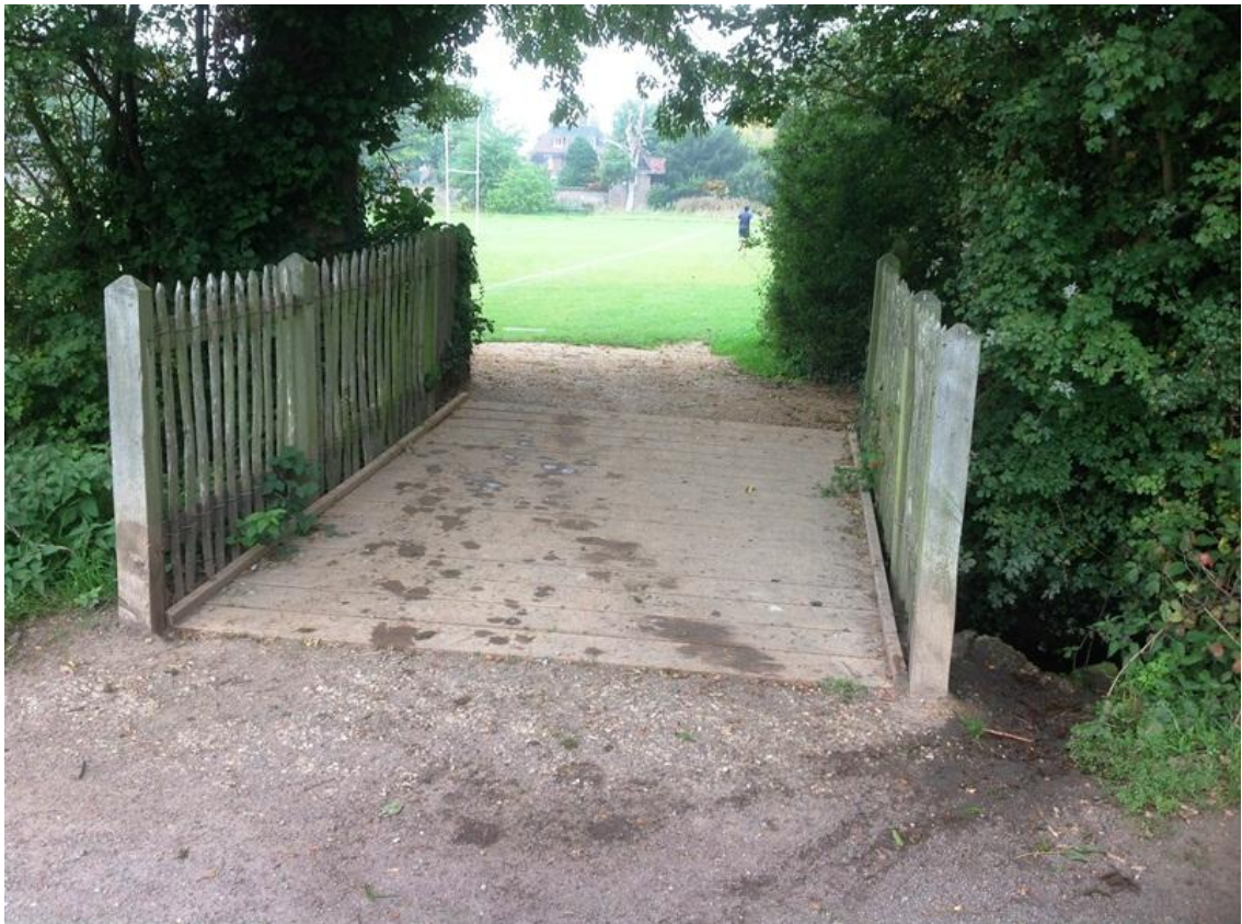
Figure 5: Refurbished timber bridge on the Heath Extension
