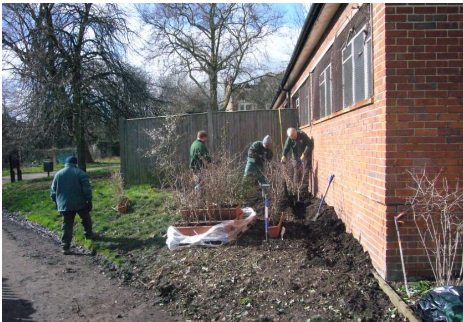
Figure 10: New oak planters in front of the Parliament Hill Café with new planting scheme
